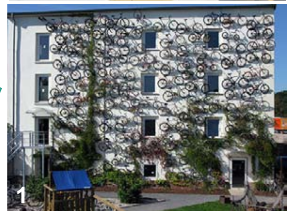
Art displays could help softening the Civic Center facade along the Arterial
