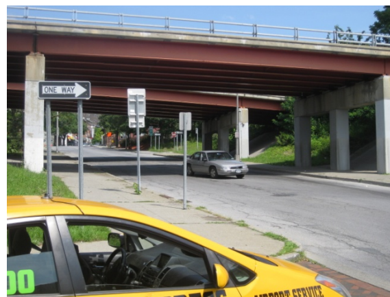
View of Rt. 9 underpass looking east on Main St.
